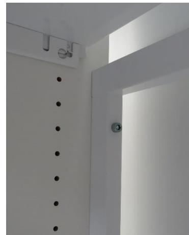
Abb./Pic. 9: Wandbefestigung / wall fixing
